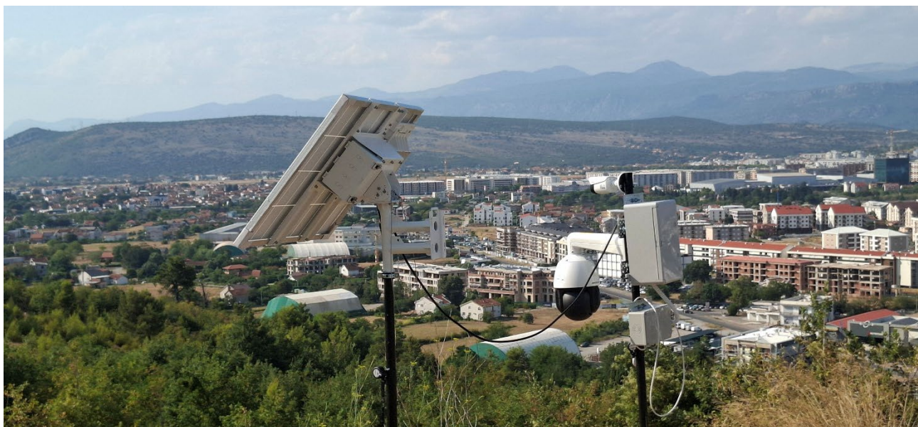
Figure 7. View of the monitored area from the Dajbabska Gora installation site overlooking Podgorica and the surrounding forested terrain.
